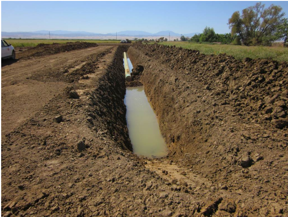
Photo 4: Buried pipe west of D-44 and east of Interstate 5.
