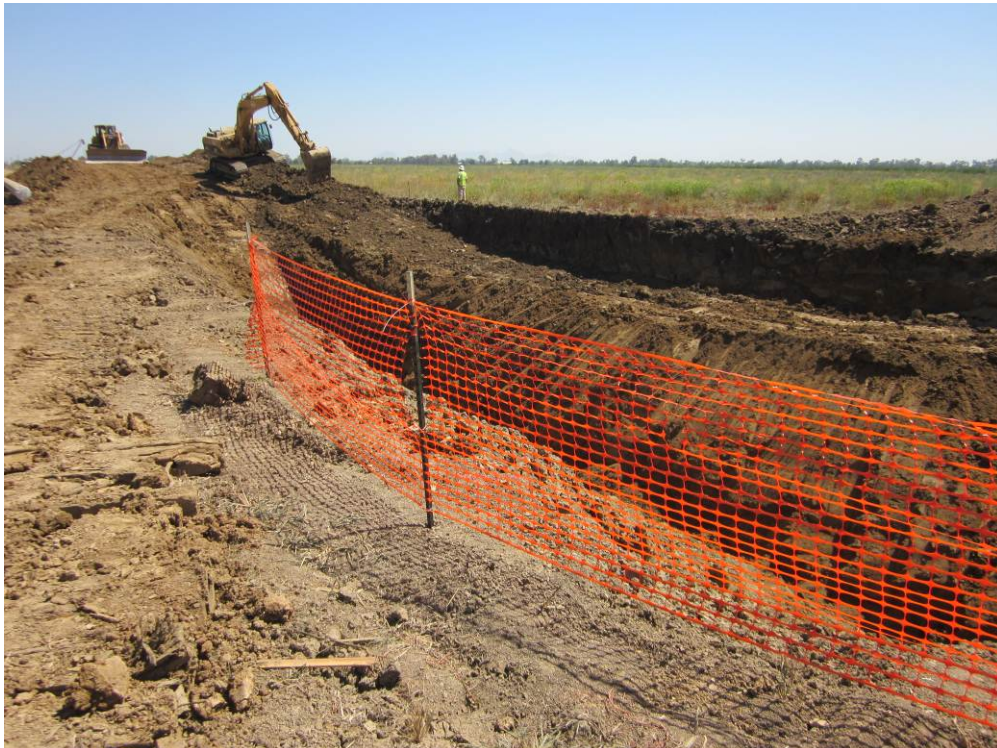
Photo 2: Auger bore hole excavation at D-25.
